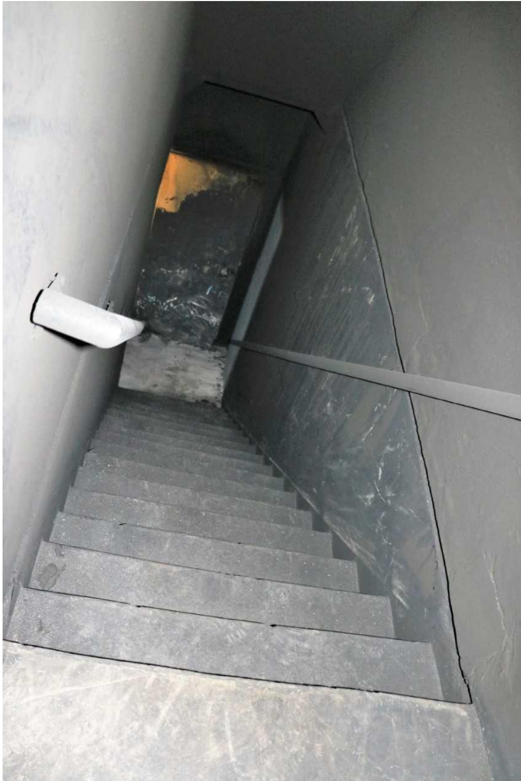
Interior Access Stairway down to Burn Room
