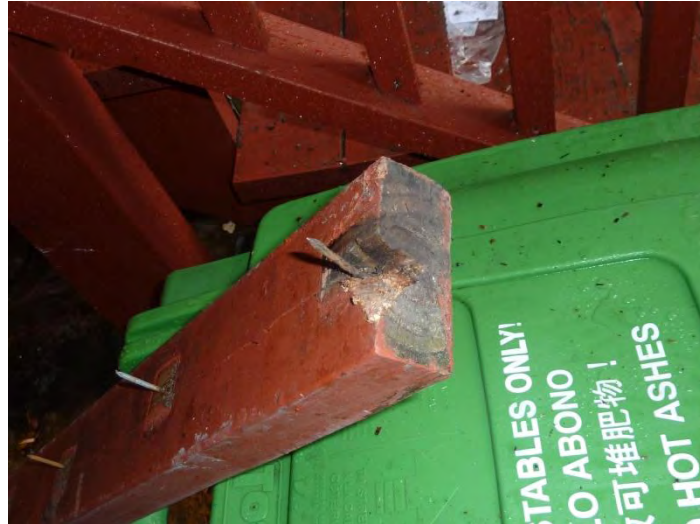
Handrail found at ground level. Note size of nails
