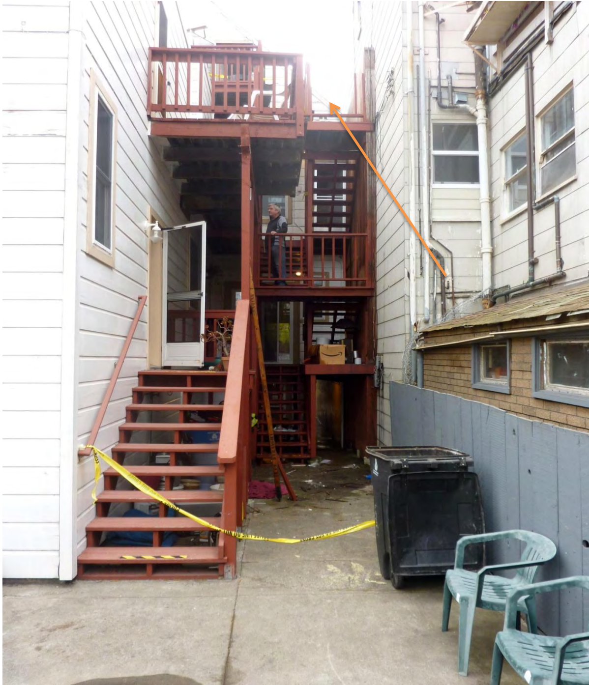
Rear deck view with arrow pointing to area of guardrail failure
