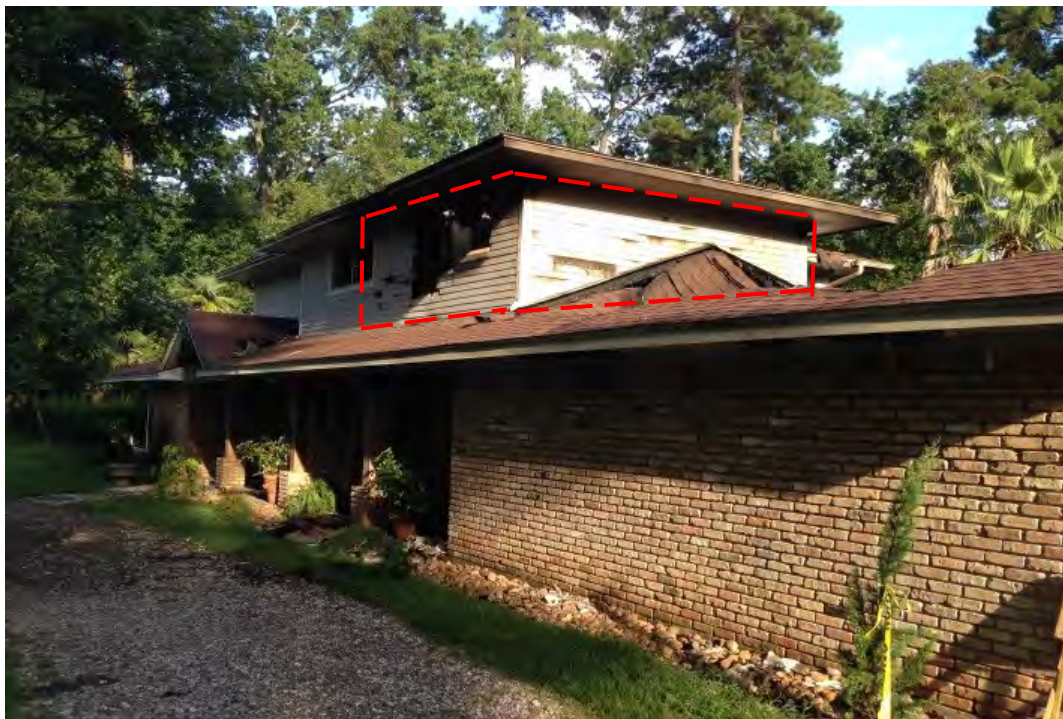
Area of void space. The garage attic opened into the void space at the garage roof peak.
